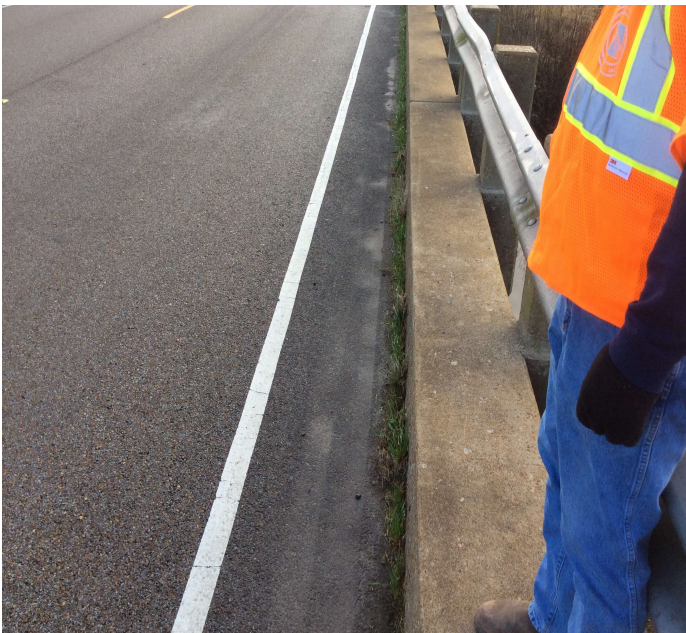
PHOTO 1 Description Vegetation is growing in gutters.
